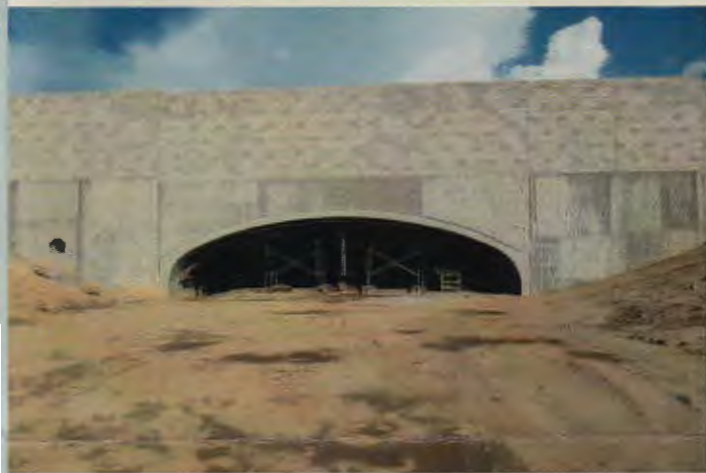
Above: This wide wildlife underpass is just south of the wildlife bridge and will provide wildlife a way to safely move under Oracle Road. Thanks to you, this important structure will soon be finished!
